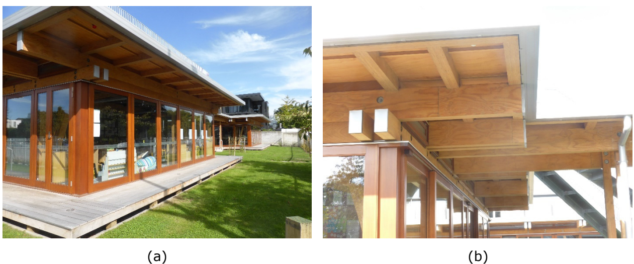
Figure 3-31: Low-rise, open floor-plan timber structure used for the Cathedral Grammar School buildings. (a) Global view, (b) Close-up view of structural detail of timber beam and columns
