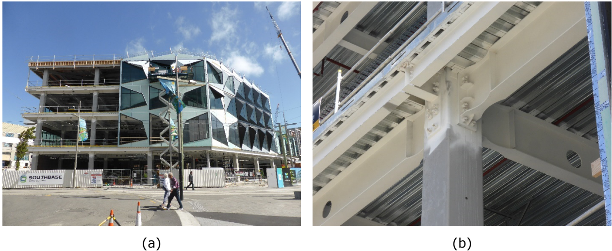
Figure 3-8: MRF at the Crossings, 71 Lichfield Street. (a) Global view of space moment frame, (b) Close-up of RBS connection with bolted end-plate to moment-resisting connection to square steel section
