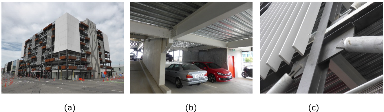
Figure 3-32: Building at 160 Lichfield Street with BRBs in one direction and structural walls in the other. (a) Global view, (b) Wall view, (c) BRB connections
