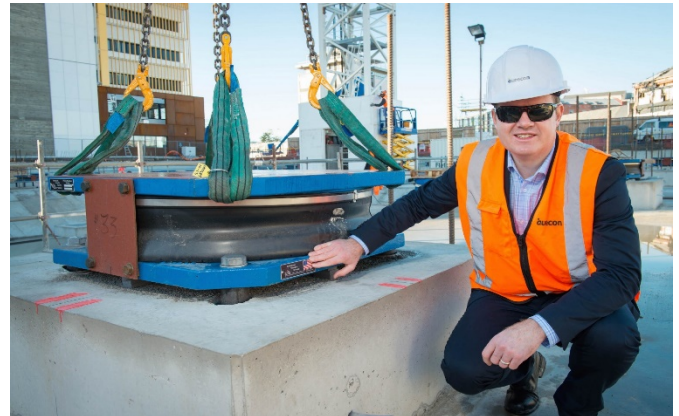
Triple Pendulum Bearing Three Seismic Isolators
