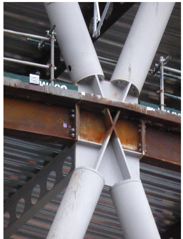
Figure 7-3: Wellington base-isolated building with exoskeleton CBF. (a) Global view, (b) Promotional information, emphasising high seismic-design level, (c) Base isolators and gap at ground level, (d) Close-up view of brace connections and floor system
