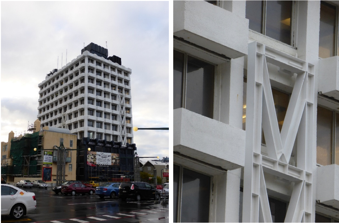
Figure 7-2: Example of Wellington building retrofitted with braced frames
