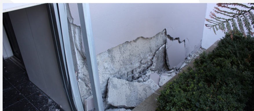
Fig 2: Web and end region crushing failures
