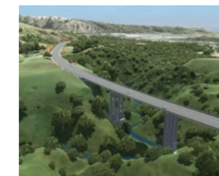
Transmission Gully Bridges to be isolated
