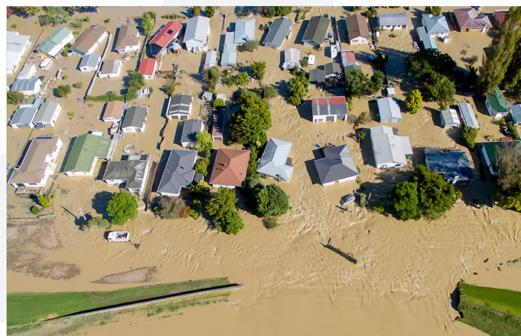
Rangataiki River stopbank breach, April 2017. Image: Sky View photography
