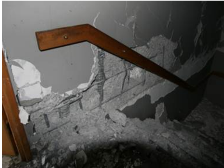
Fig. 2. An example of metal duct connection damage during the 2010/2011 Canterbury earthquakes.
