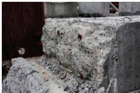
Figure 4 - Cone breakout failure observed during panel demolition
